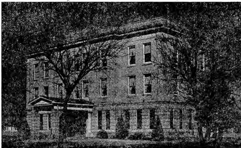
TO BE TORN DOWN — The St. John's Junior School pictured here will be torn down to make room for the new million dollar stadium, a spokesman for the Board of Trustees announced last Friday. Bryan, Robinson, and Walker Demolition Co. has contracted to raze the building. School officials estimate that it will take them only a short while to do the job.
